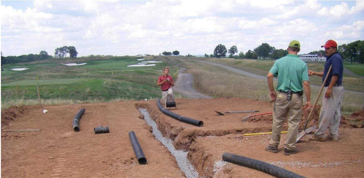
*Figure 4. Drainage installation during the construction of a new tee. Photo credit: Thomas Turner.*
